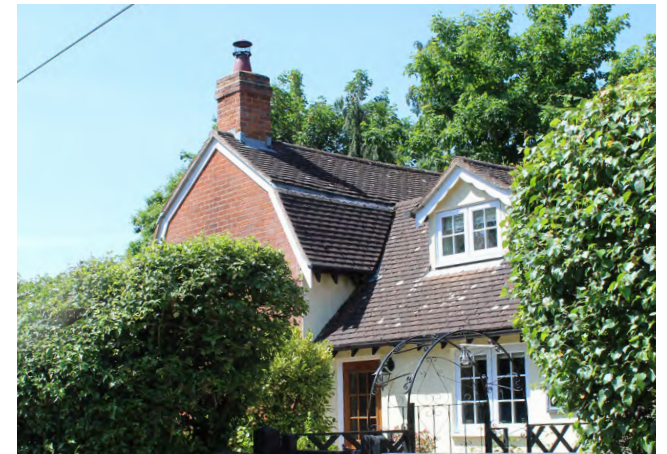
Figure 44: Churnwood Cottage on Chapel Lane, with a gambrel roof and decorative bargeboarding
