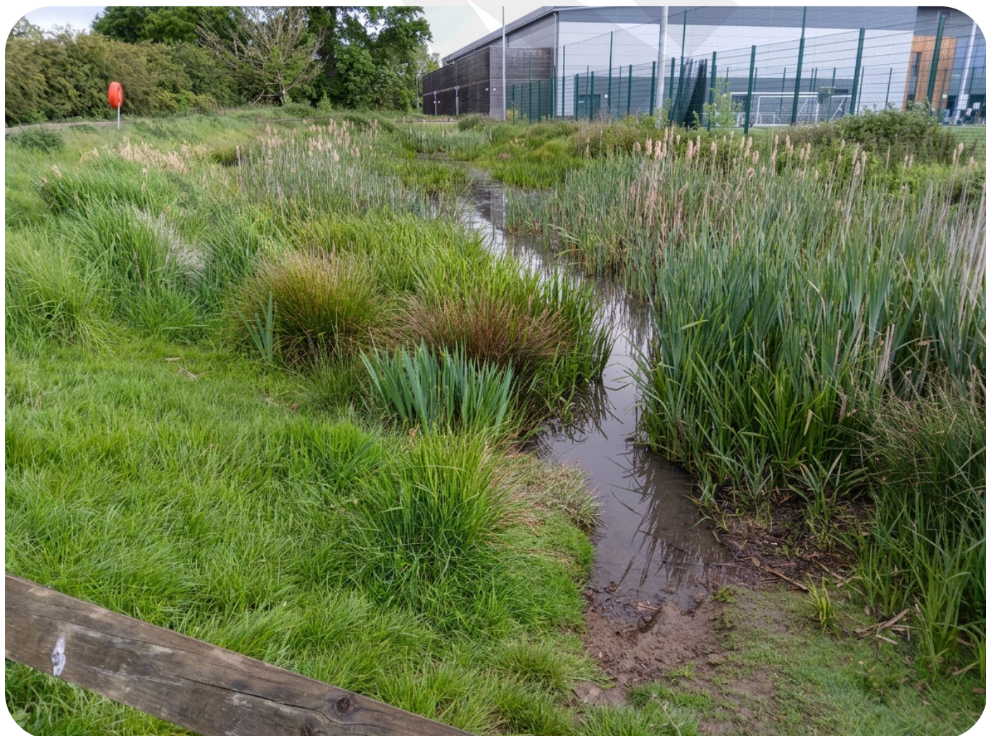
Figure 4 - Photo SuDS measures. Attenuation basin at Braywick Leisure Centre
