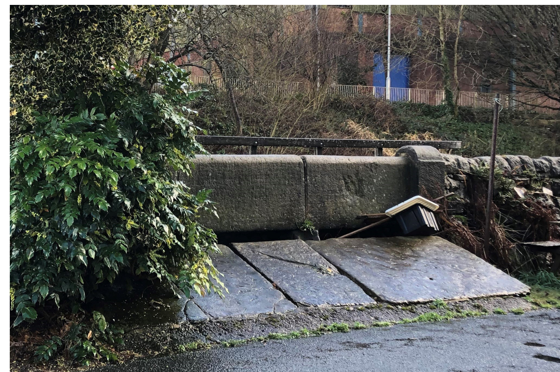
4. Apron & Lower weir covered by inclined stone slabs (Comercial St. view).
