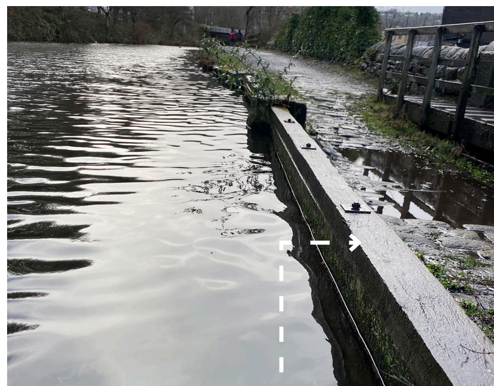
5. Side weir and washwall - currently leaking water.
