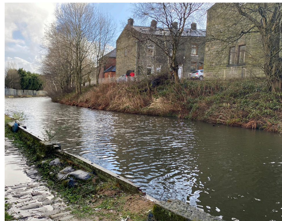
2. Rochdale Canal - showing existing weir in disrepair with sandbags.
