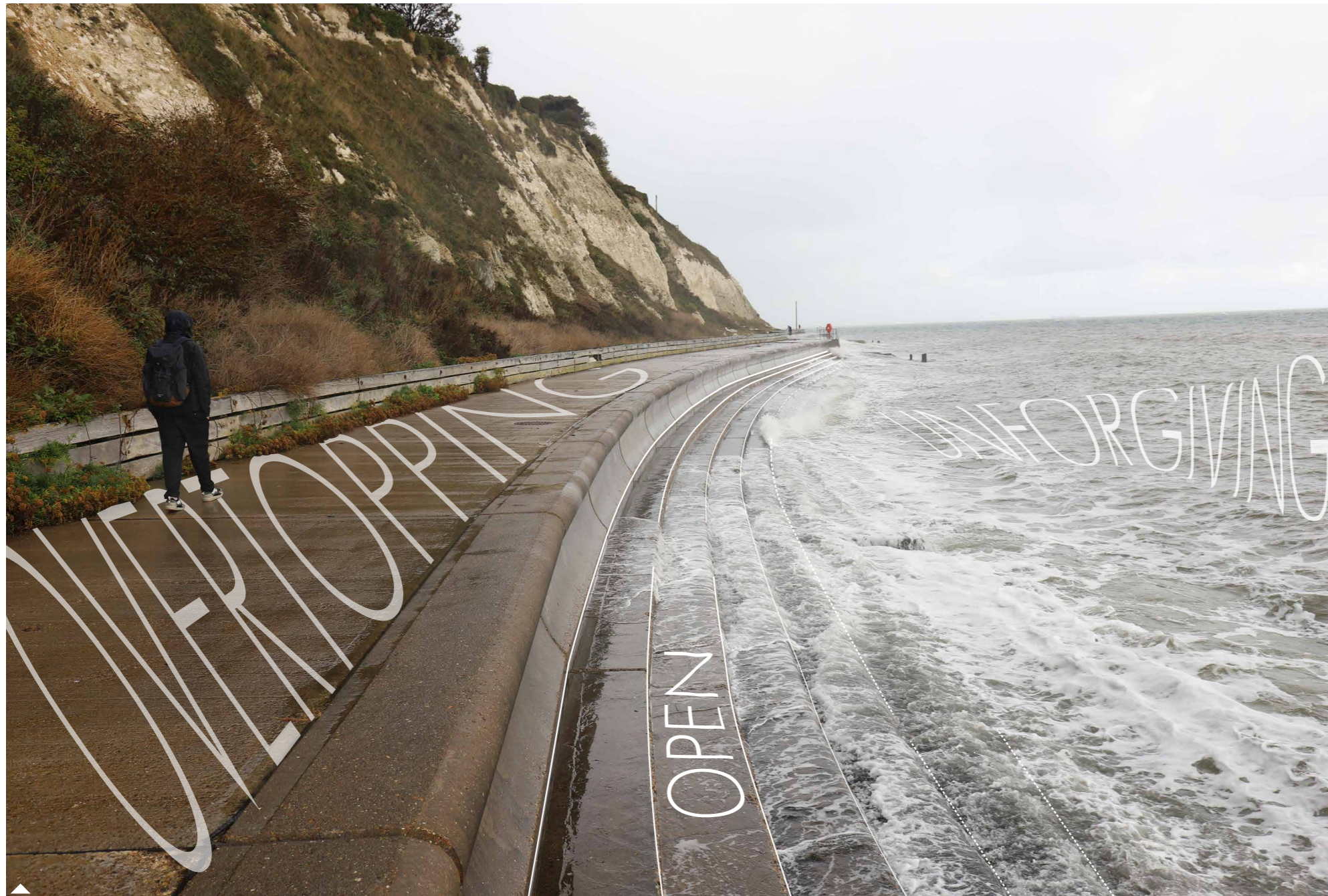
View from the promenade / concrete stepped revetment looking east, north-east along the sea defences towards the headland to Horseshoe Bay | Photo taken at high tide.
