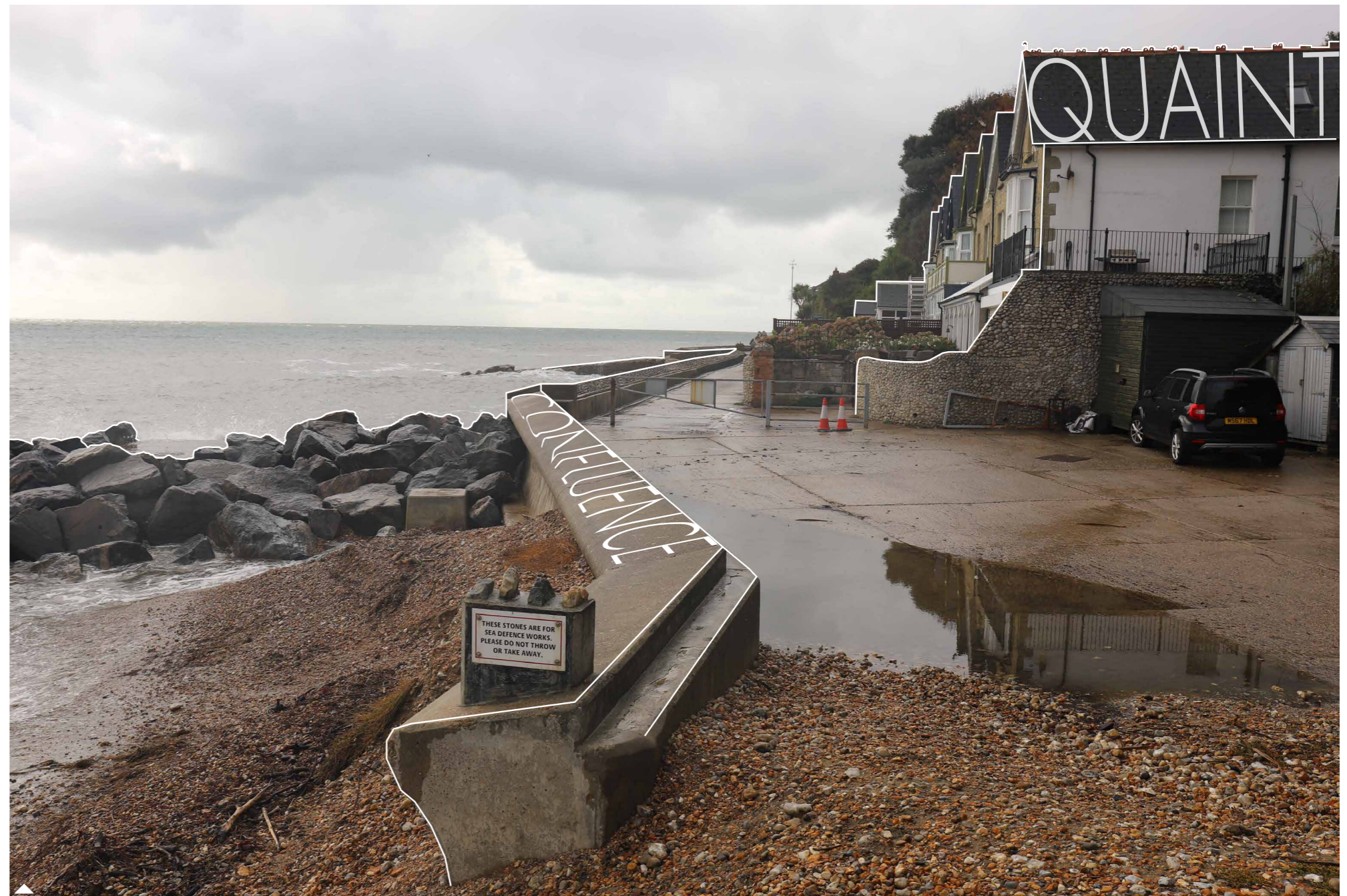
View from the western extent of Monks Bay beach looking south west along the sea defences | Photo taken at high tide.
