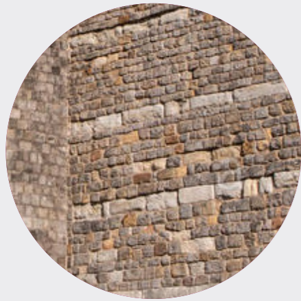
Historic sandstone within castle wall with natural variation in texture and tone
