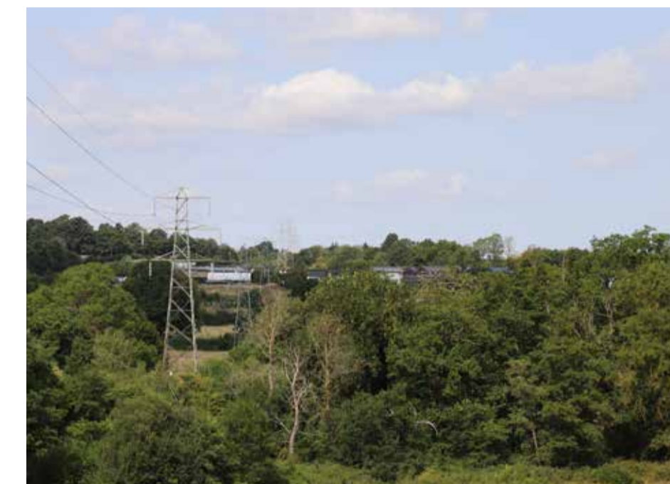
2 Above-ground pylons to the north
