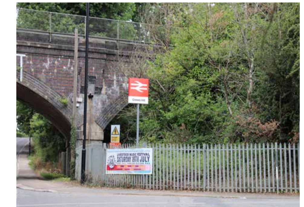
7 Viaduct at entrance to Crews Hill station
