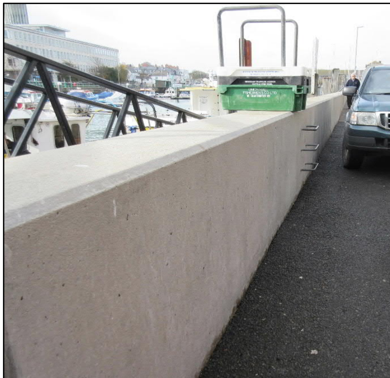
Figure 3.2 Typical existing 'Harbour Sea Defence Wall' (Wall 7, adjacent to Lifting Bridge abutment)
