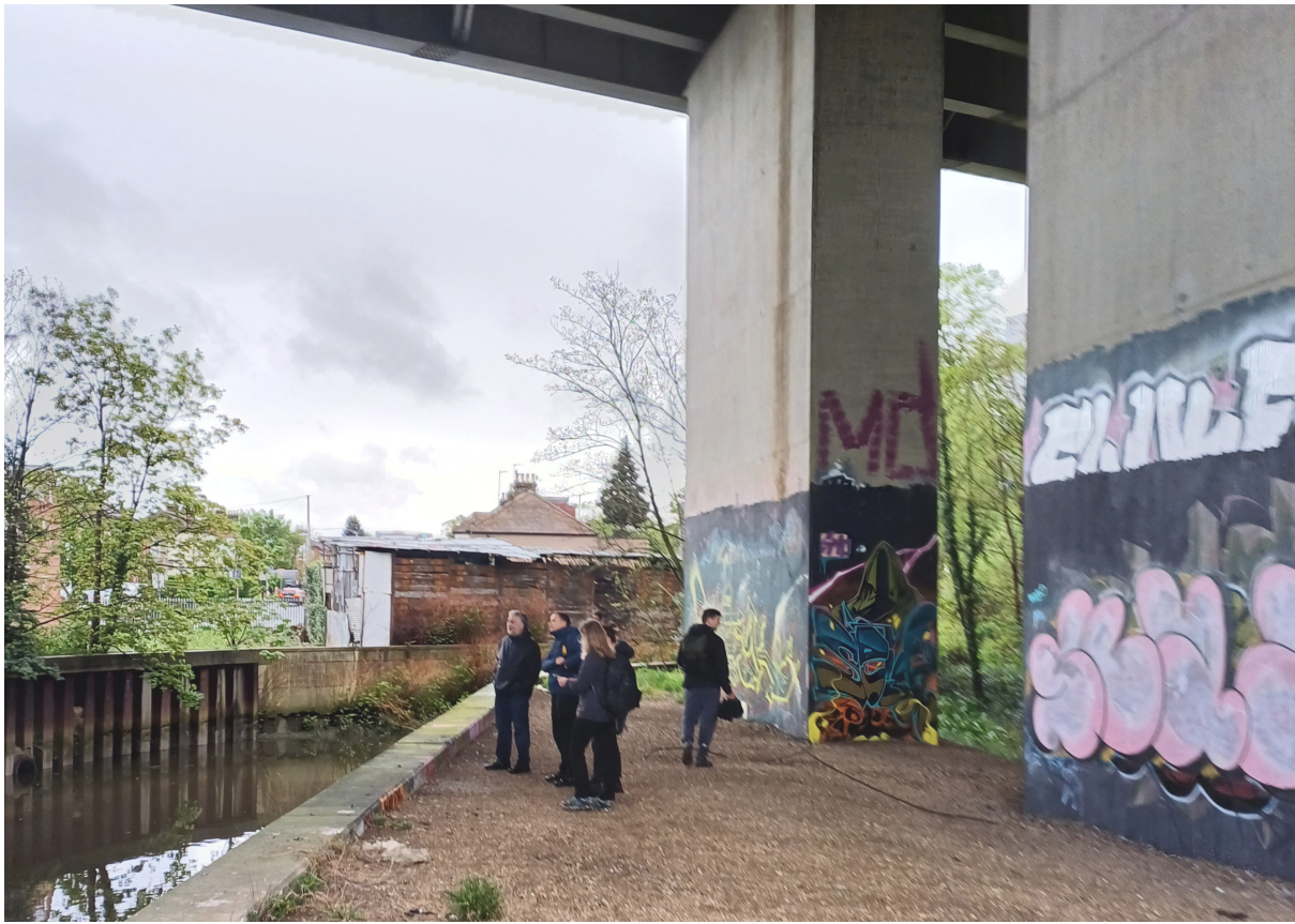
Existing condition underneath A406 flyover
