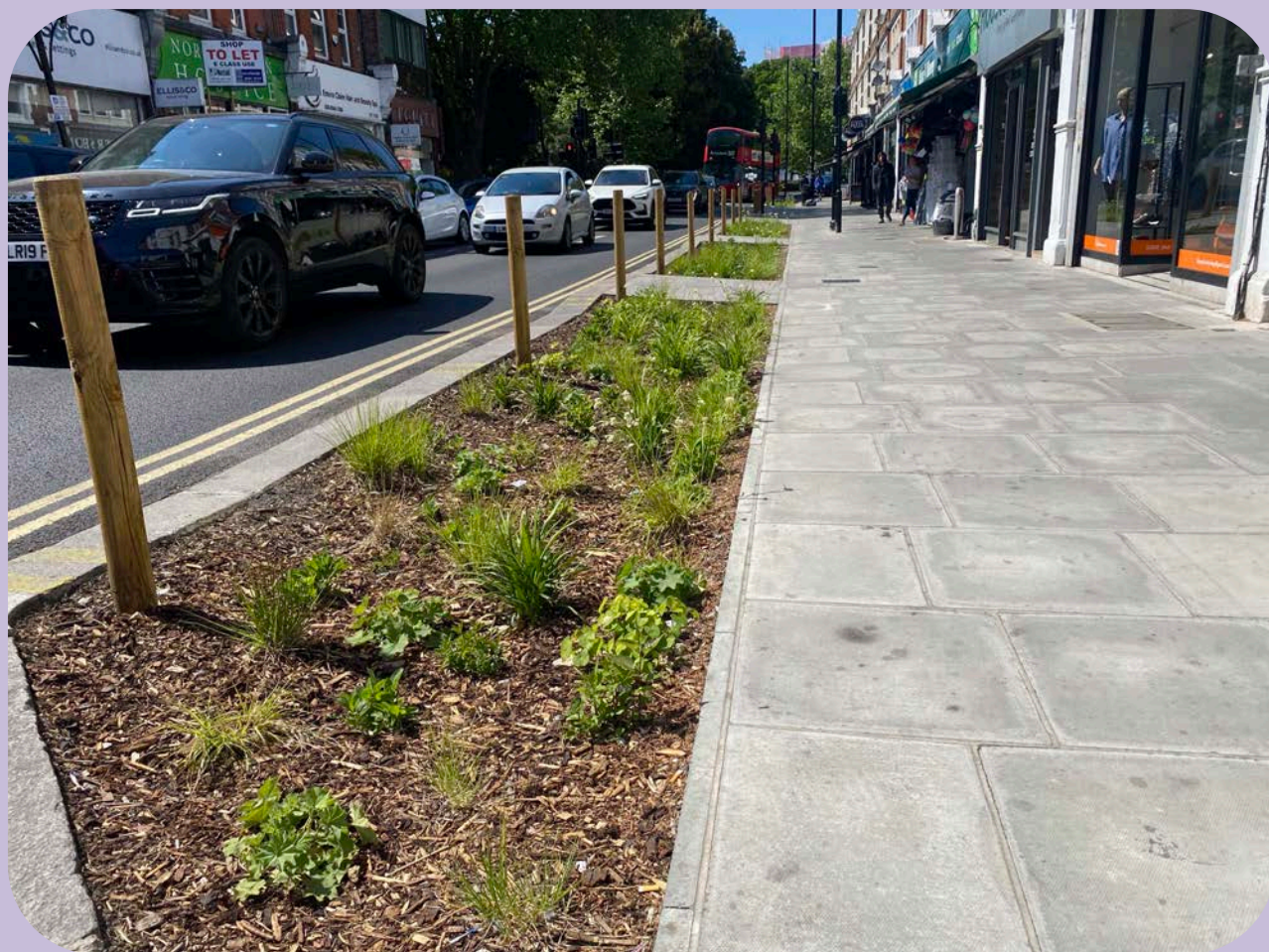
New rain gardens installed as part of Phase 1
