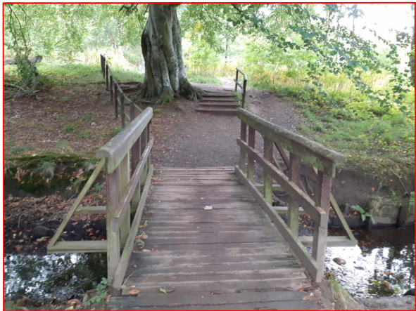
Existing wooden bridge to be replaced with a new 6m long, 1.8m wide, recycled plastic, wood-effect, bridge. Steps to be renewed and an additional step provided to ease gradients
