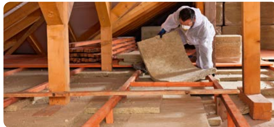
A person installing loft insulation.
