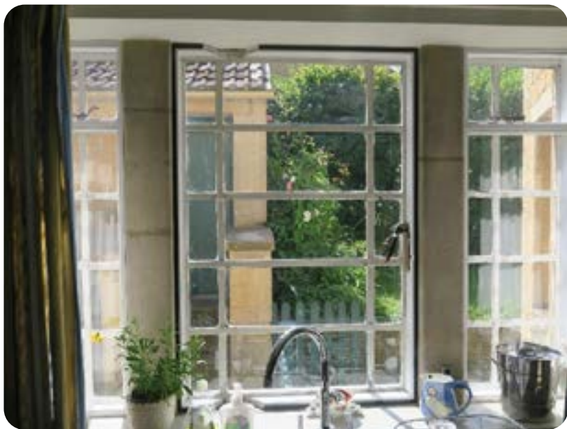
Photograph of secondary discreet glazing on metal frame window. Credit (Bath Preservation Trust)
