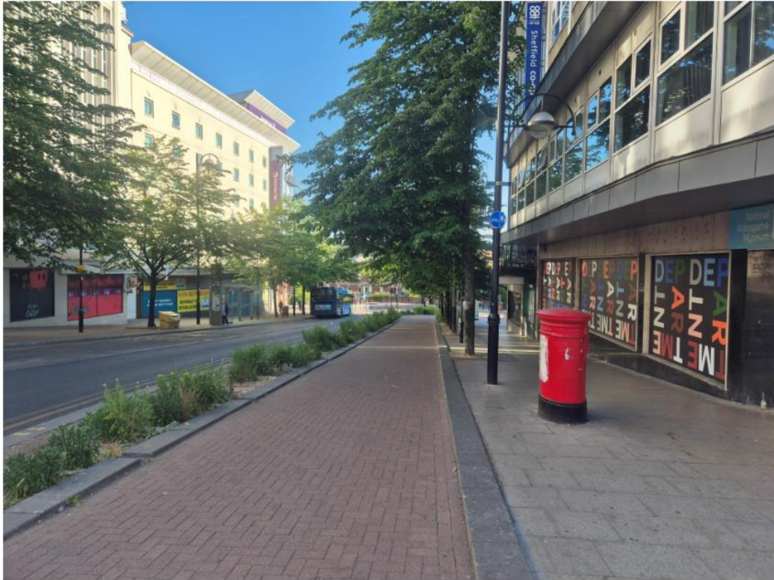
Nearby Angel Street which shows the standard of materials we will upgrade Castle Street to
