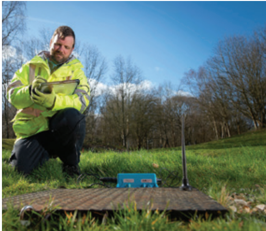
Butler Water Treatment Works, Kent
