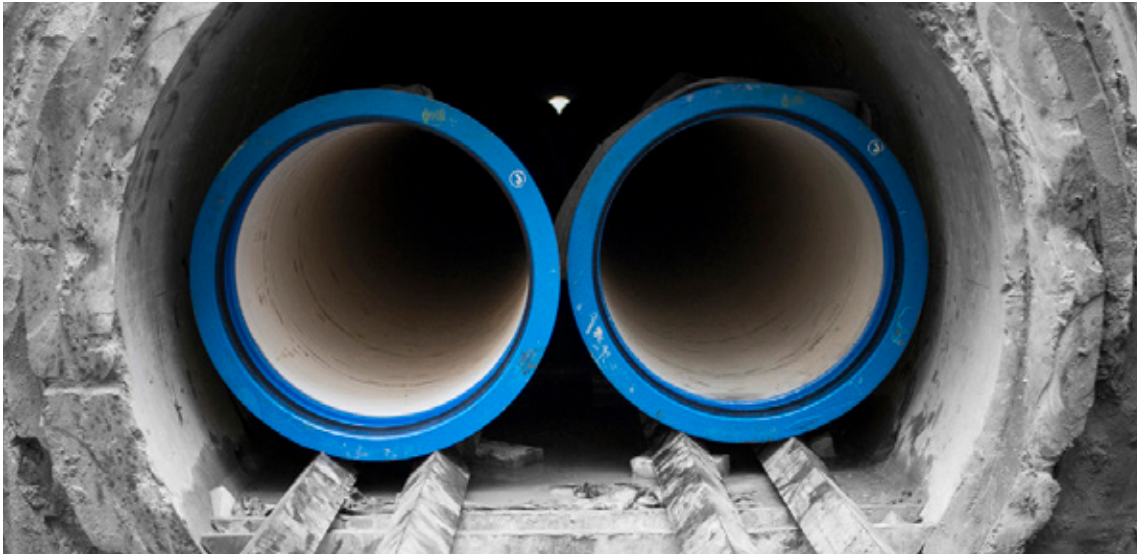
Laying a two strategic water pipelines in at Aylesford, Kent
