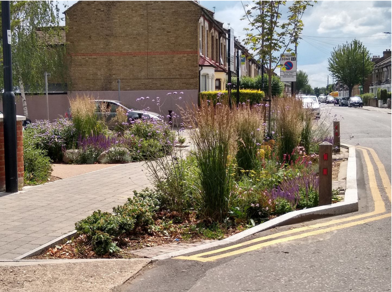
Award winning rain garden scheme which uses planted build outs to help traffic calming, Haselbury in Enfield delivered by Enfield Council.
