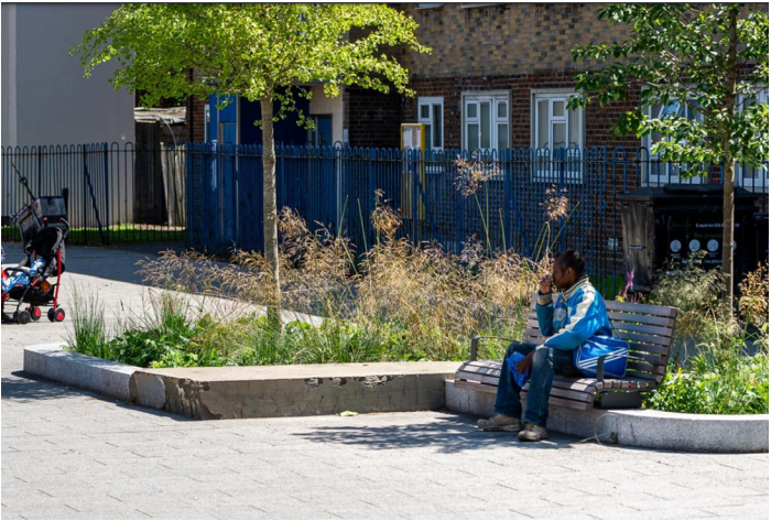
Example of rain gardens at White Hart Lane using kerbs and boulders with gaps between for water infiltration
