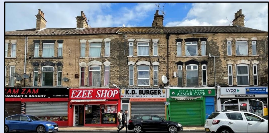
Figure 58 - Photograph towards 100-112 Spring Bank (north) (Author, 2023)
