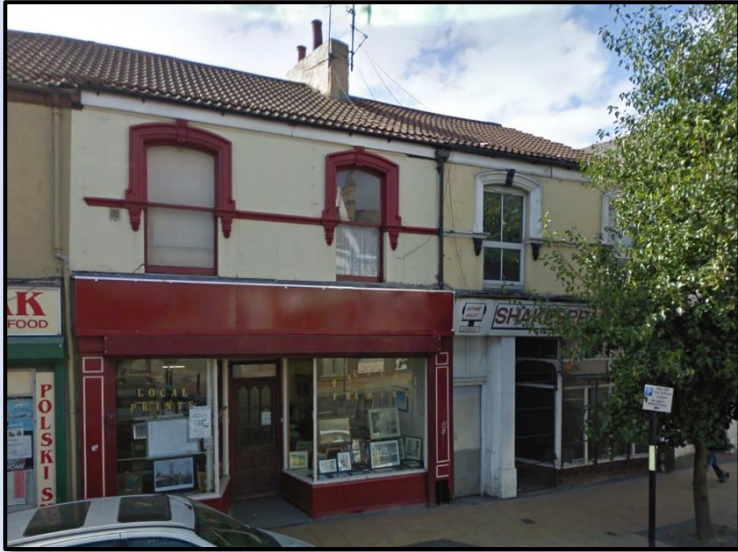
Figure 104 - 173-175 Spring Bank in 2009 (after designation) with the original shopfronts still in-situ with the recessed central/side entrances (the pilasters and corbel details to No 173 are a later addition and the fanlights have been concealed). (Google Maps, 2009)
