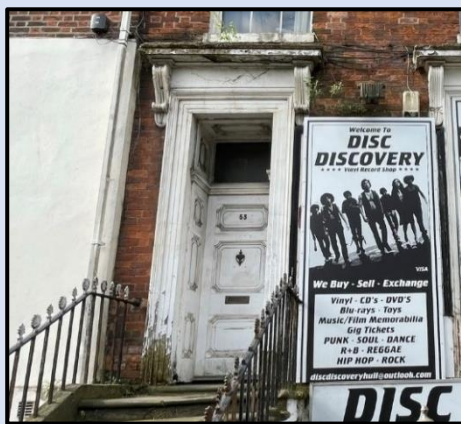
Figure 93 - Original doorway entrance and portico with scroll details and plaster surround (Author, 2023)
