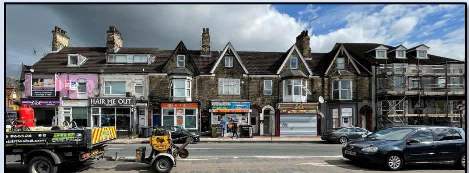
Figure 44 - Photograph of 230 to 246 Spring Bank (north) (Author, 2023)
