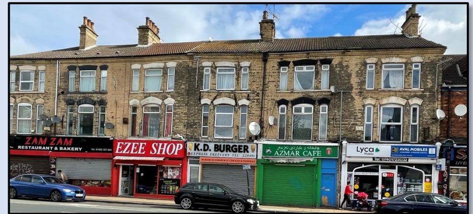
Figure 127 - 104-110 Spring Bank showing the lack of care in the shopfront design and general maintenance that reduces the quality of the buildings from positive to neutral buildings (Author, 2023)
