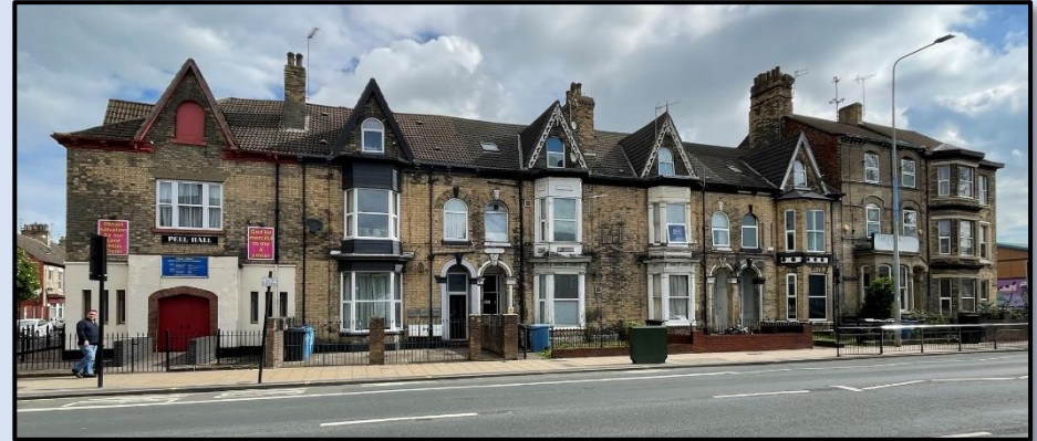
Figure 43 - Photograph of 136 to 148 Spring Bank (north) (Author, 2023)
