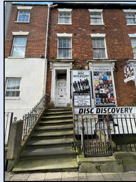
Figure 84 - Stone steps leading to the elevated ground floor residential entrance providing privacy to the primary living space. (Author, 2023)
