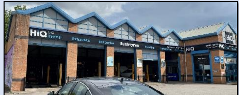
Figure 68 - The Hi-Q garage to the north side of Spring Bank which is set back from the dominant building line to provide sufficient turning areas for vehicles (Author, 2023)
