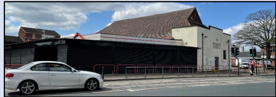
Figure 130 -Retail unit that extended the former Church Hall to St Jude's Church creates a negative frontage and lacks quality (Author, 2023)
