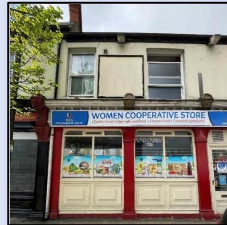
Figure 101 - 171 Spring Bank has retained its historic shopfront but has suffered from intrusive signage and loss of decorative corbels. (Author, 2023)
