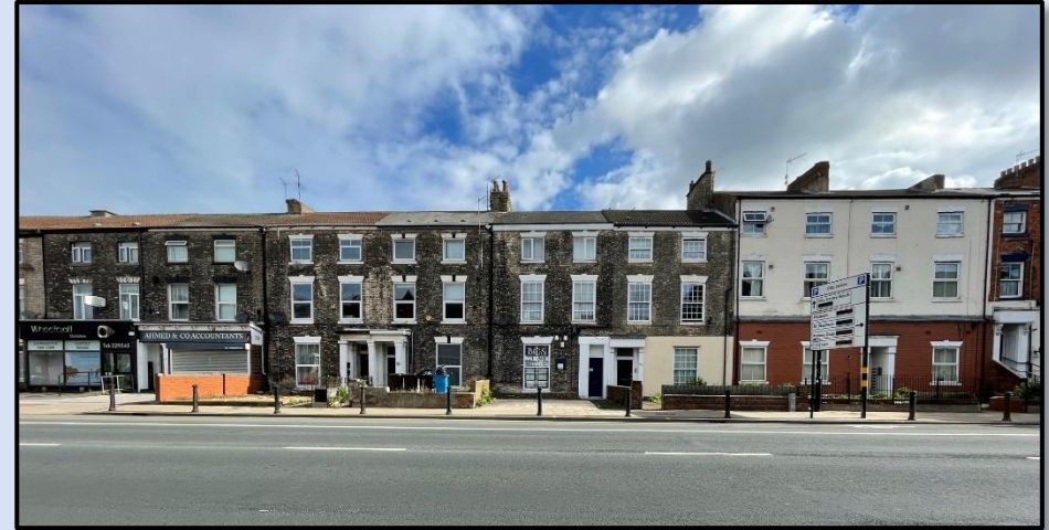
Figure 21 - Photograph of 58 to 72 Spring Bank (north side) (Author, 2023)
