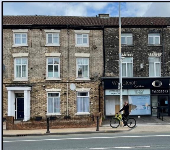
Figure 73 - The use of buff brickwork to the Georgian buildings dating from pre 1830. (Author, 2023)
