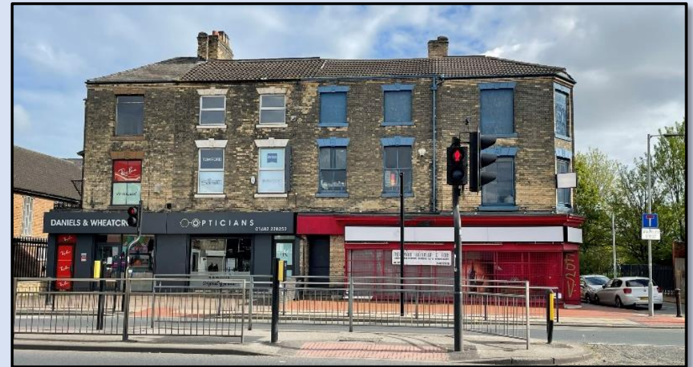
Figure 142 - Spring Bank elevation of 84-90 Spring Bank from the Park Street approach (Author, 2023)
