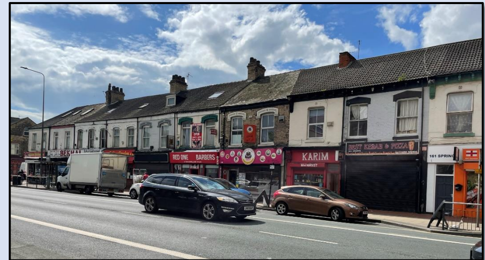
Figure 35 - Example of retail units to ground floor with residential above to the south side of Spring Bank (Author, 2023)
