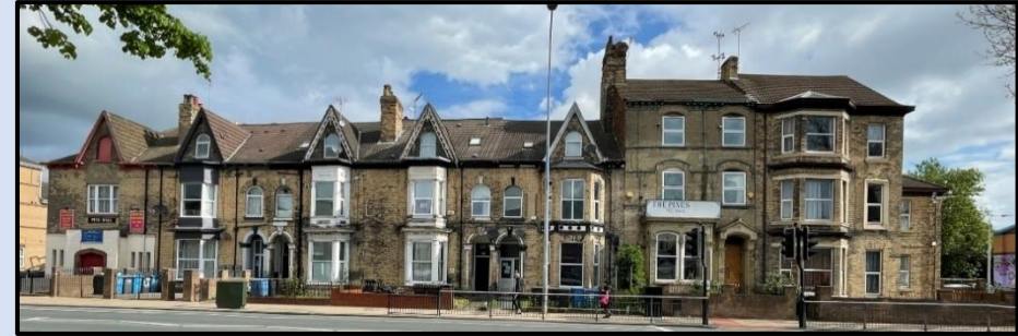
Figure 55 - Photograph towards 136-148 Spring Bank (north) (Author, 2023)
