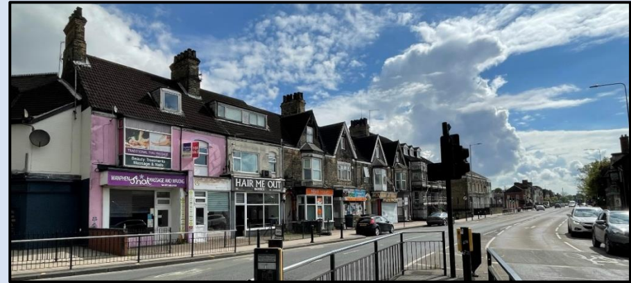
Figure 148 - View looking down Spring Bank from the north-west entrance (Author, 2023)
