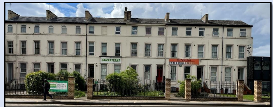
Figure 56 - Photograph towards 69-79 Spring Bank (south) (Author, 2023)
