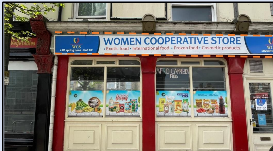
Figure 110 171 Spring Bank showing how the fascia sign is the correct depth but extends over the corbel detail (Author, 2023)
