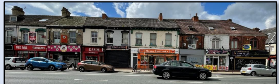
Figure 48 - Photograph towards 147-167 Spring Bank (south) (Author, 2023)
