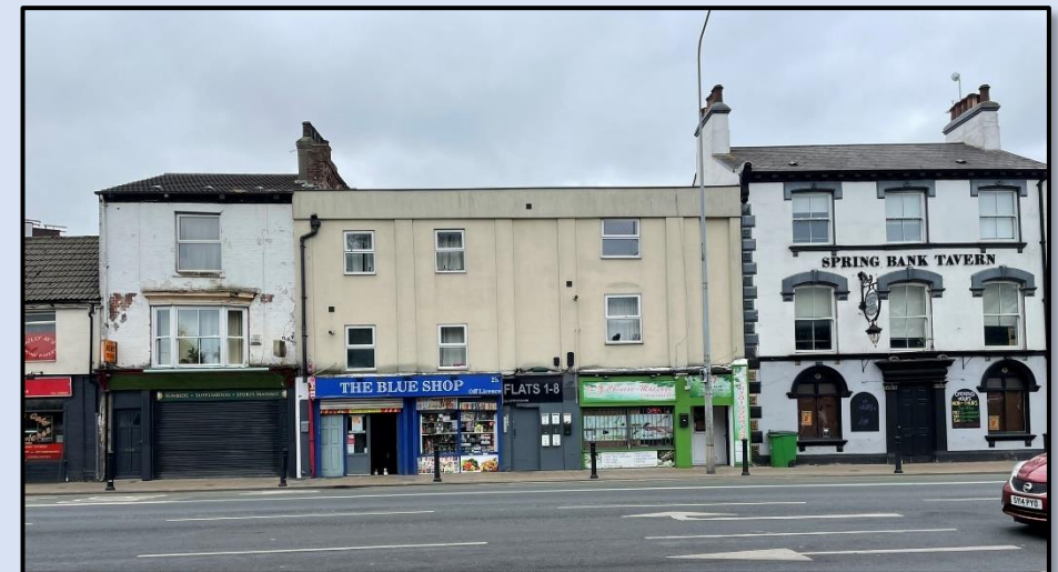
Figure 20 - Photograph towards the buildings along the south of Spring Bank, zone 1 including the Spring Bank Tavern. (Author, 2023)
