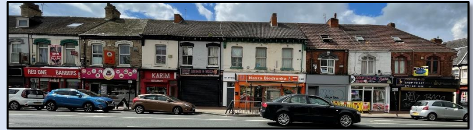
Figure 128 - 147-165 Spring Bank showing the lack of care in the shopfront design and general maintenance that reduces the quality of the buildings from positive to neutral buildings (Author, 2023)
