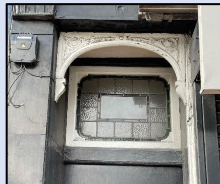
Figure 79 - Cast iron arched doorway detail and decorative fanlight retained (Author, 2023)
