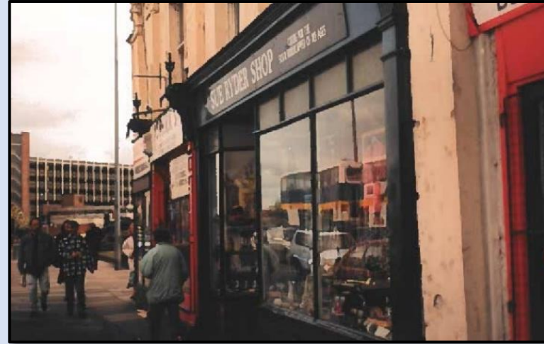
Figure 102 - 19 Spring Bank in 1995 shortly before Conservation Area Designation with the traditional shopfront retained including the recessed door and fanlights (Hampel, 1995)
