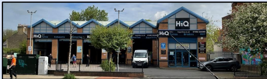
Figure 57 - Photograph towards 124-134 Spring Bank (north) (Author, 2023)
