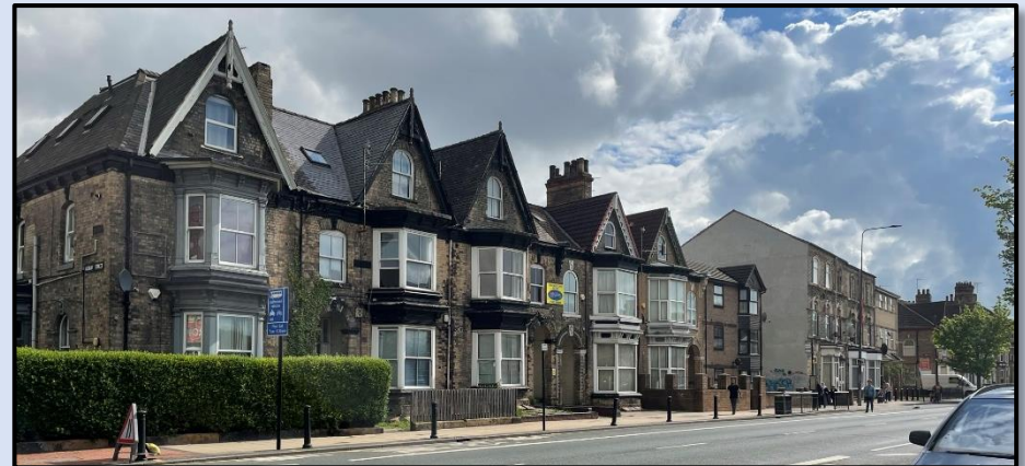
Figure 45 - Photograph of 150 to 168 Spring Bank (north) (Author, 2023)
