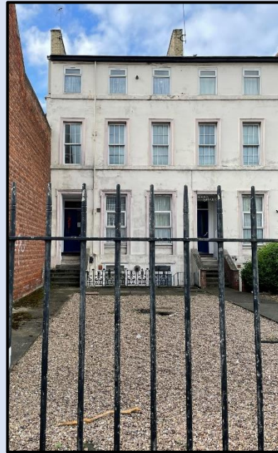
Figure 85- Modern railings installed in the 1980's to form the boundary of 69-79 Spring Bank (Author, 2023)
