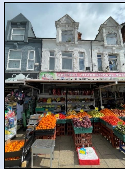
Figure 61 - Photograph towards 198 Spring Bank (north) (Author, 2023)
