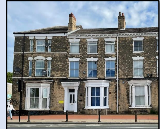
Figure 82 - Pitched roof with limited detail at roof level with the exception of the timber gutter supports. (Author, 2023)
