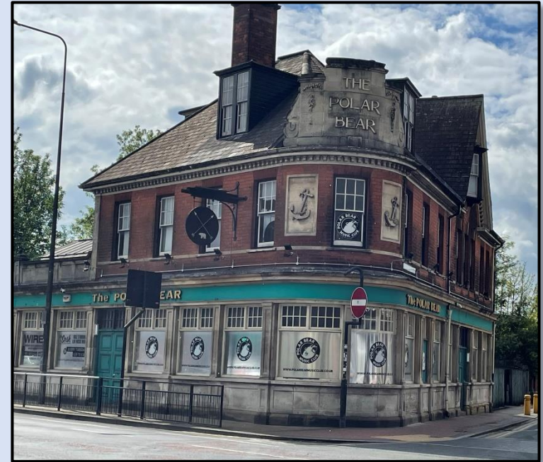
Figure 80 - The roof form of the Polar Bear which curves at the corner, allowing the buildings form to turn the corner. (Author, 2023)
