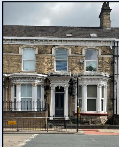
Figure 75 - The use of buff brickwork to the Late Victorian buildings towards the west of Spring Bank. (Author, 2023)
