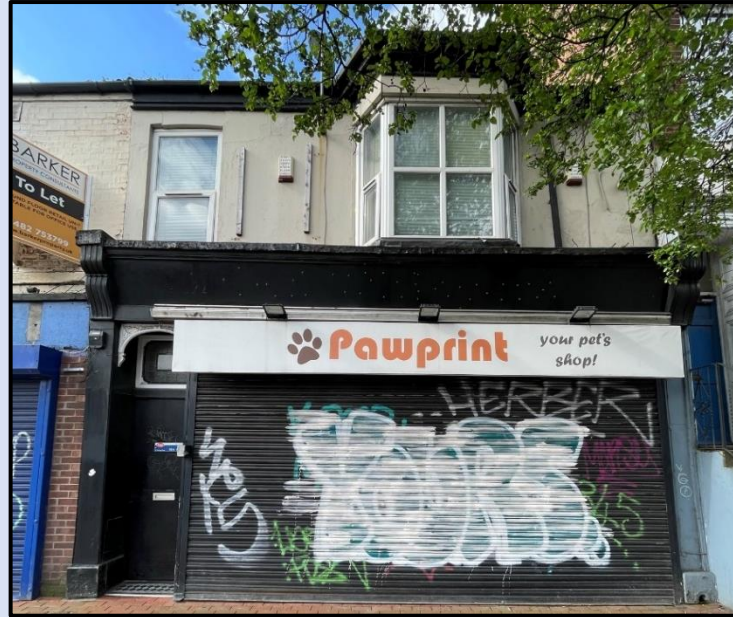
Figure 95 - Pawprints unit which has retained its original cornice, fascia, pilasters and doorway details. (Author, 2023)
