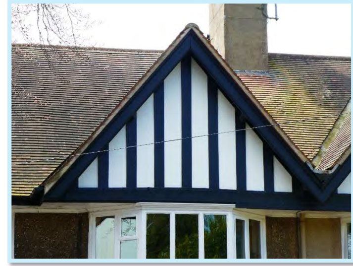
Figure 26 Close stud 'Mock' panelling.
