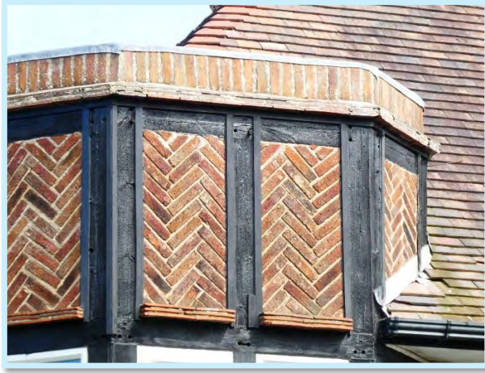
Figure 24 - Herringbone Brickwork at No.45.
