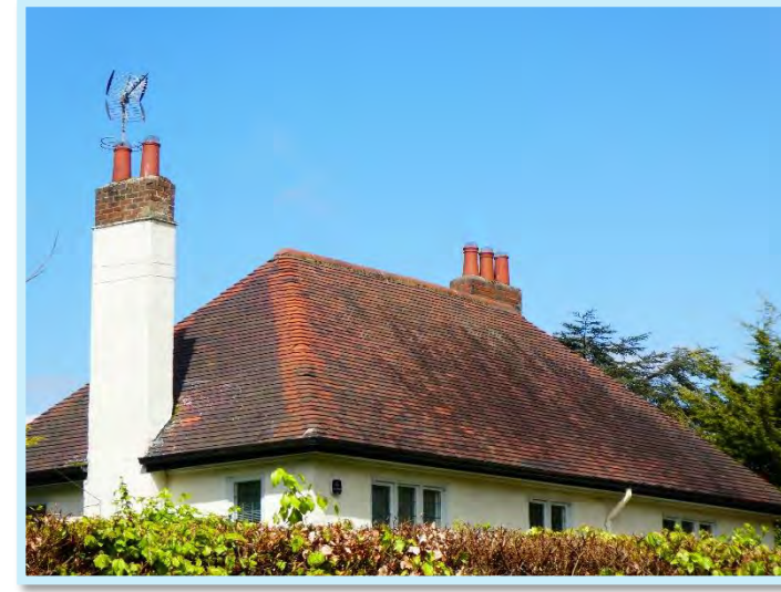
Figure 17 Hipped roof and clay tiles at No.90.
