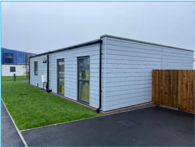
1: Prefabricated Home Constructed for Temporary Accommodation, Cardiff. Daiwa Homes, @Home, Beattie Passive
