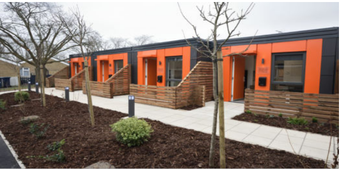
3: Prefabricated Home Constructed for Temporary Accommodation, Cambridge, UK, Solohaus
