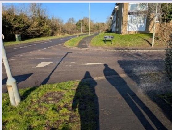
Figure 8: Lack of tactile paving on crossing over side roads of Upavon Way
