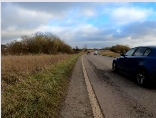
Figure 46: Cyclists have to use the small gutter verge, whilst the carriageway is very wide meaning cars travel at high speeds
