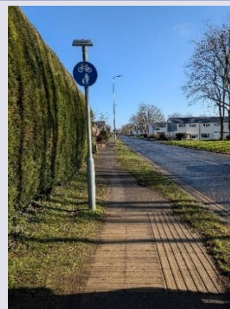
Figure 11: Unclear/ incorrect signage and tactile paving indicating a shared use footway/ cycleway
