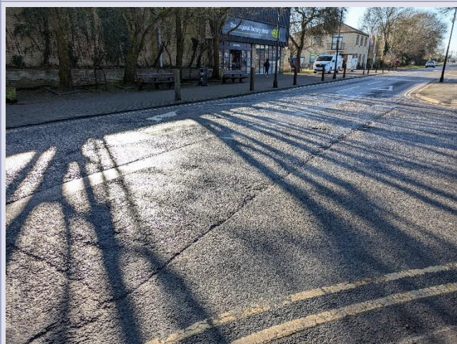
Figure 32: Unclear markings showing the mini roundabout make pedestrian movements difficult and unsafe
