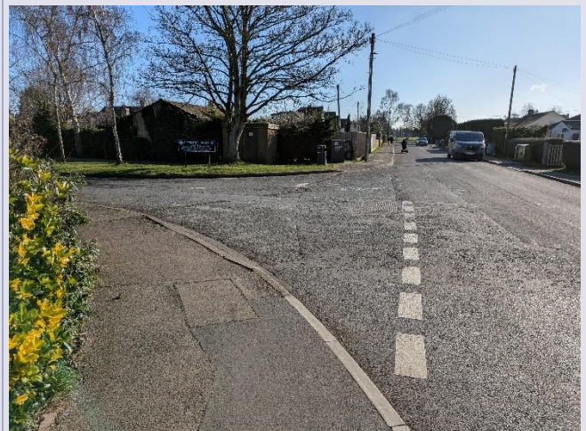
Figure 35: Junction of Swinbrook Road and Glenmore Road very wide and missing tactile paving on dropped kerbs
