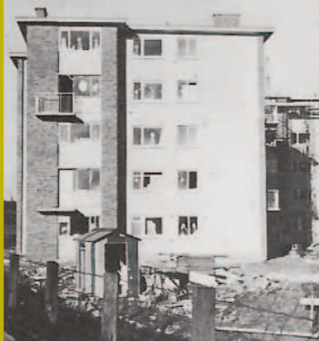
Redburn View West, 1958
